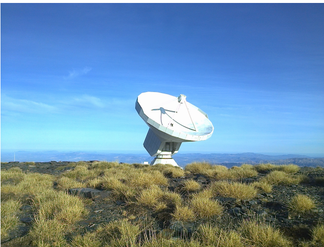
Figure 5: The fully steerable IRAM-30m telescope (Cassegrain design).
