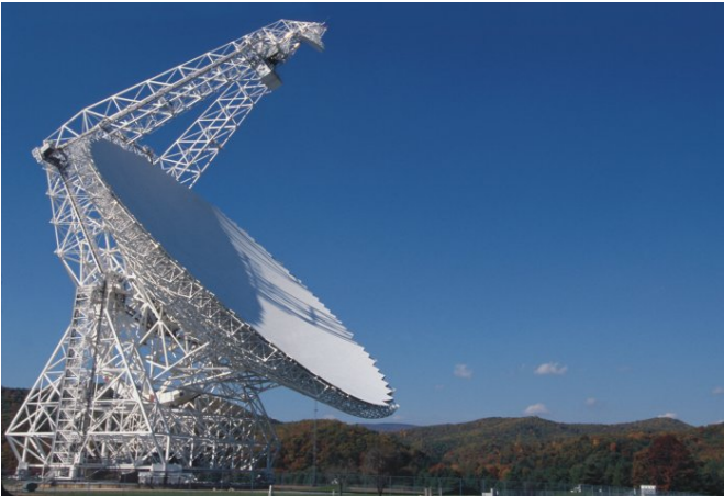
Figure 4: The fully steerable Green Bank 100m telescope (Gregorian, off-axis; active optics).
